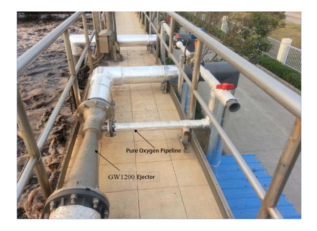
Factory photo of secondary injection efficiency device
